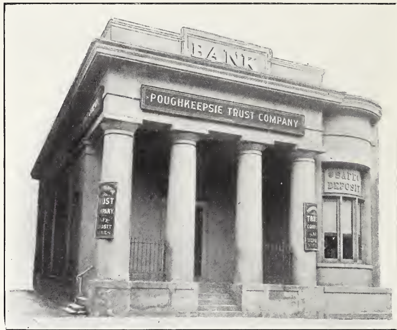
Poughkeepsie Bank Building, now the Poughkeepsie Trust Company, (see Appendix). The addition to the right was recently built.
